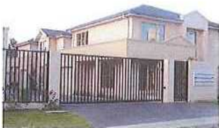
1800mm High Steel Palisade Security Fence
